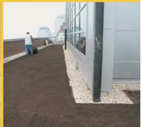
Spreading and compressing the soil.
