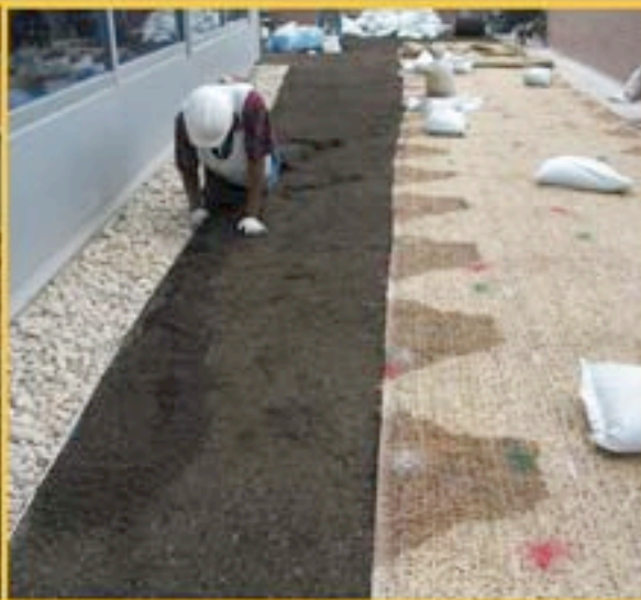
Covering with more soil and laying out a biodegradable coconut fiber mat.
