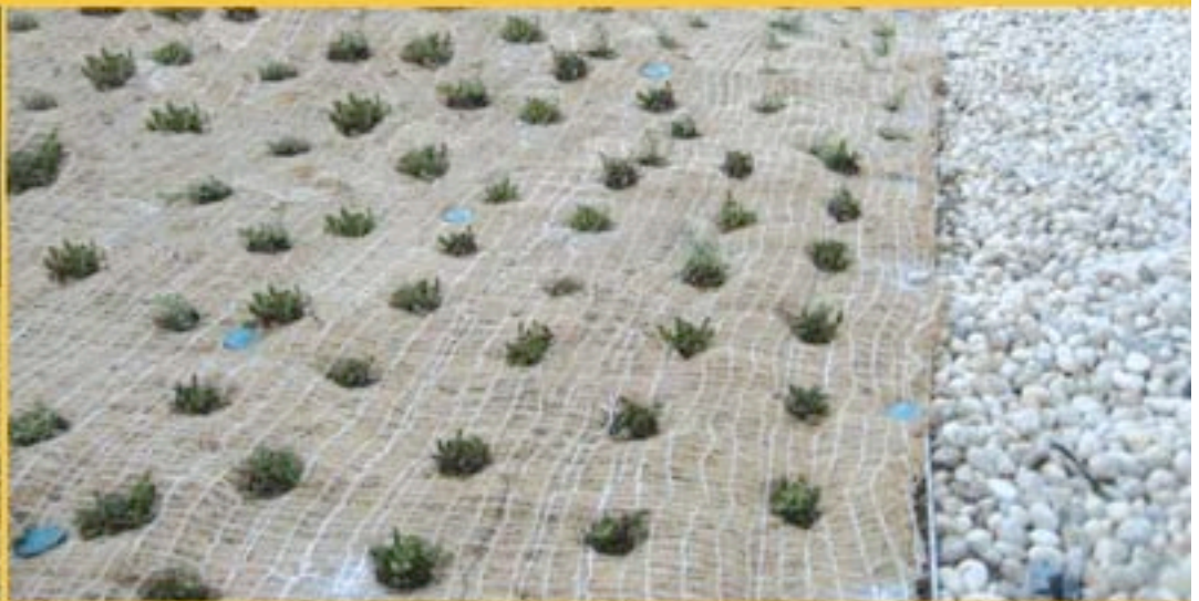
Over time the coconut mat will disintegrate as the sedums grow and their roots develop a stronger grip into the soil beneath.
