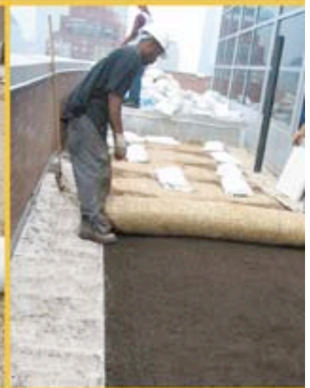
Covering with more soil and laying out a biodegradable coconut fiber mat.
