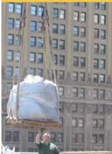
Hoisting the soil, the gravel ballast, and all other material.
