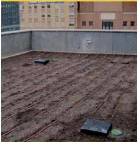
Laying out a temporary irrigation system.
